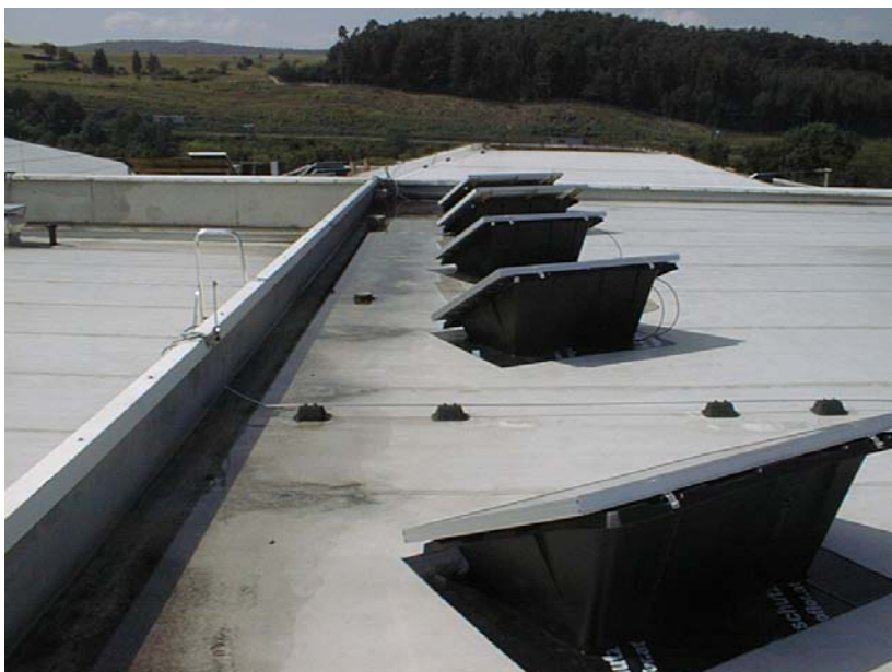
Fig. 2: Example for mounting on ConSole, Ubbink Solar
