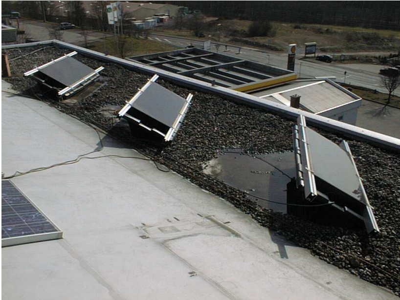
Img. 3: Even at flattish positions of the sun there is no shadow
