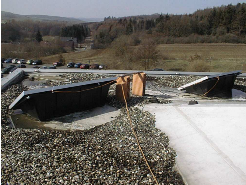
Img. 5: Both SCHOTT panels oriented west displayed from behind
