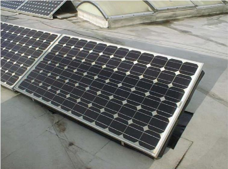
Fig. 6: example of row-by-row shading
