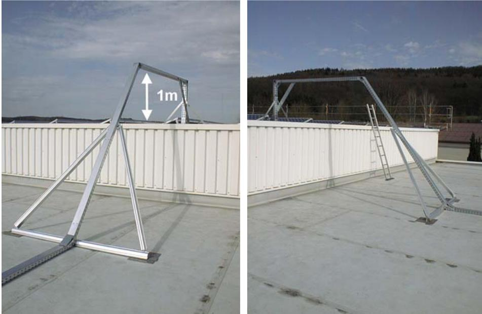
Fig. 7a, 7b: Bridging of the parapet while keeping the required distance.
