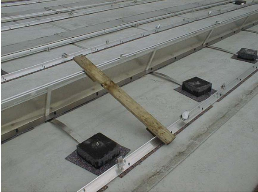
Fig. 3: Low ballast flat roof mounting system during installation.
