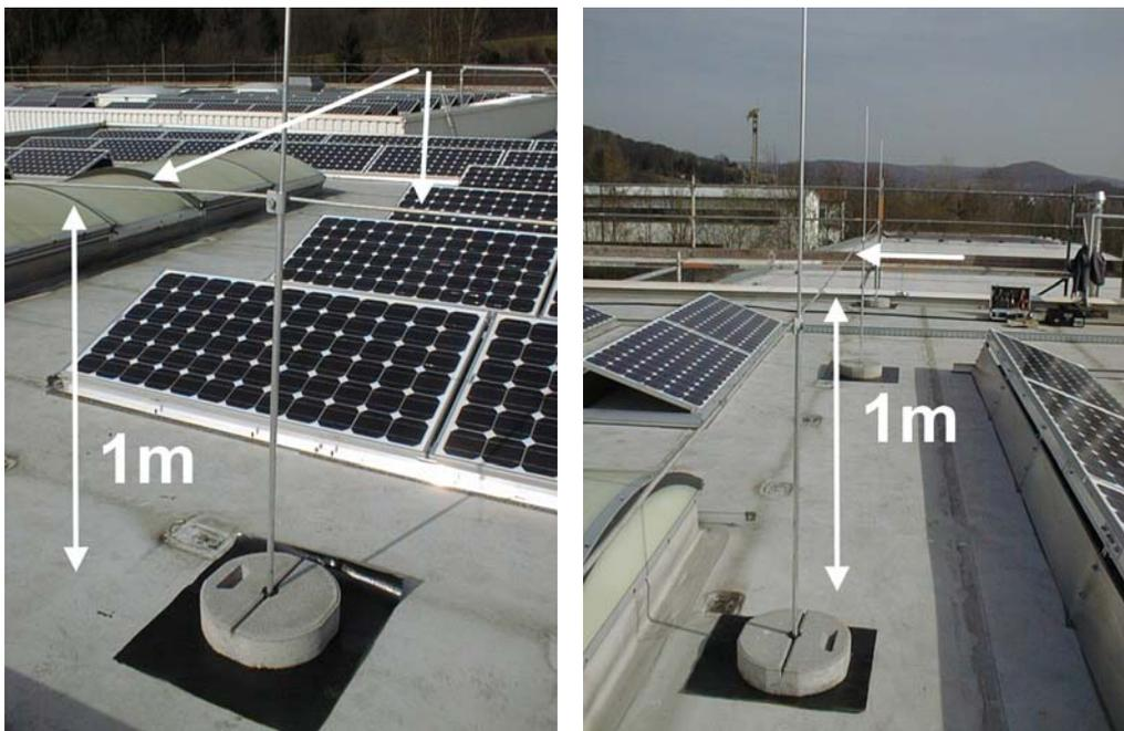
Fig. 9, 9a: Elevating a meshed conductor belonging to the air-termination system 1m above the roof
