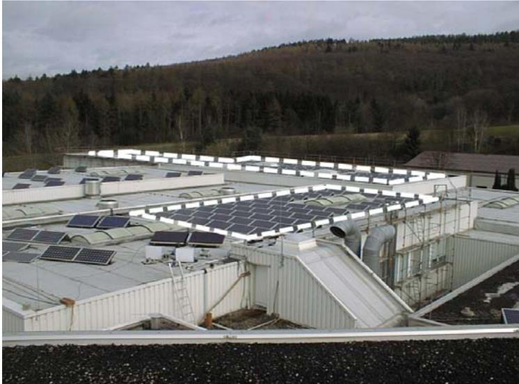
Fig. 11: completed PV system, nominal power 40kWp
