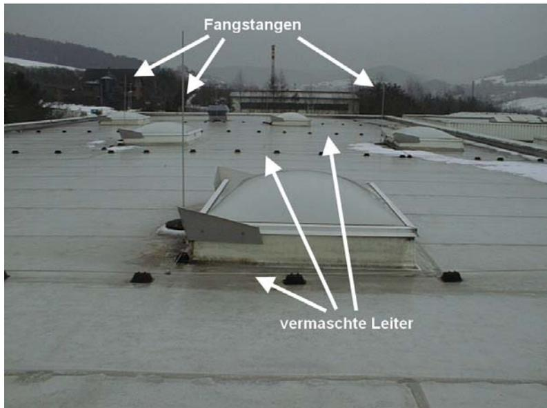
Fig. 2: roof lights, air termination rods, air-termination system (meshed conductors)
