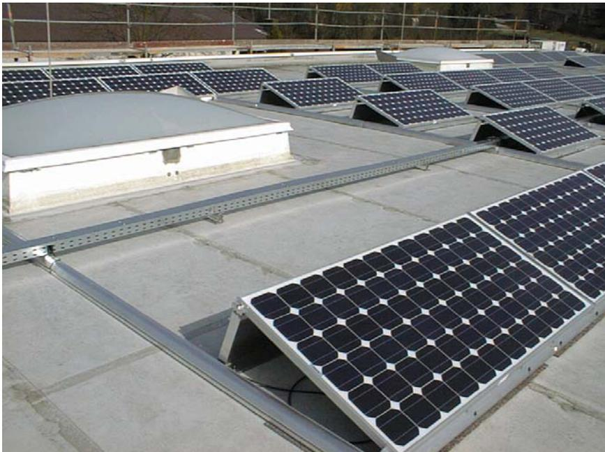
Fig. 4: Wiring inside the module frame and the cable trough.
