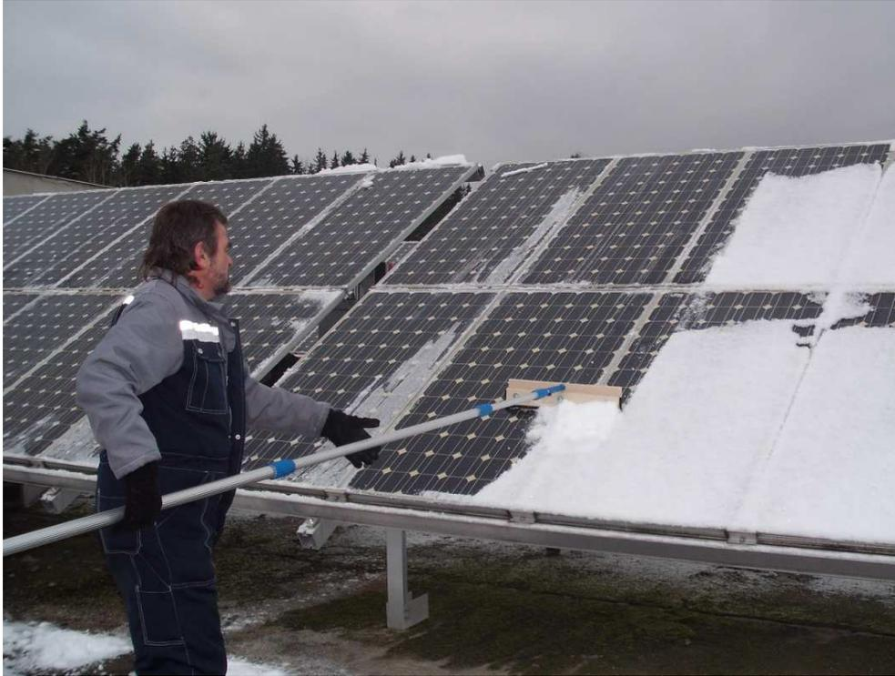
*Fig 2: Maintenance worker clearing snow with appropriate tool.*
